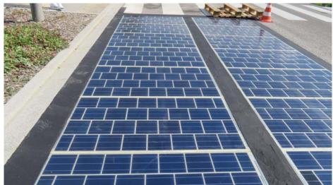
Solar panels on the road – for charging the electrical cars in movement.
